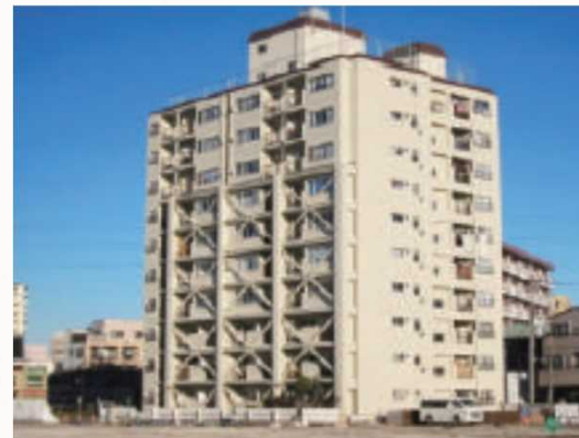
After seismic retrofitting work
