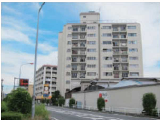
Before seismic retrofitting work
